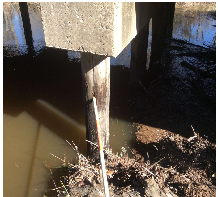
PHOTO 2 Description M0229 pile 5 bent 5 beginning to mushroom.
