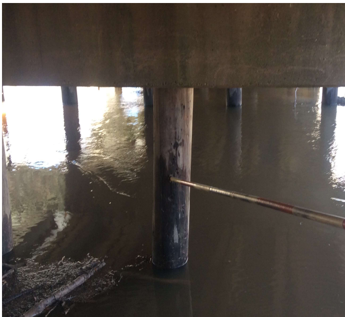
PHOTO 3 Description M0229 pile 2 Bt 5 rotten.
